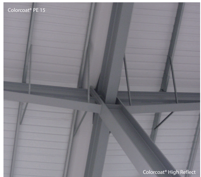
Close up showing transition from Colorcoat® PE 15 to Colorcoat® High Reflect.
